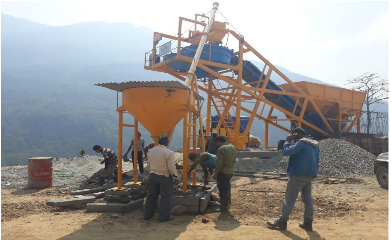
Fig:-Batching plant being installed at suitable location
