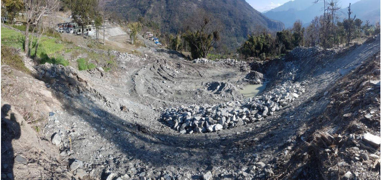
Fig:-Site clearance and excavation work at Surge Shaft
