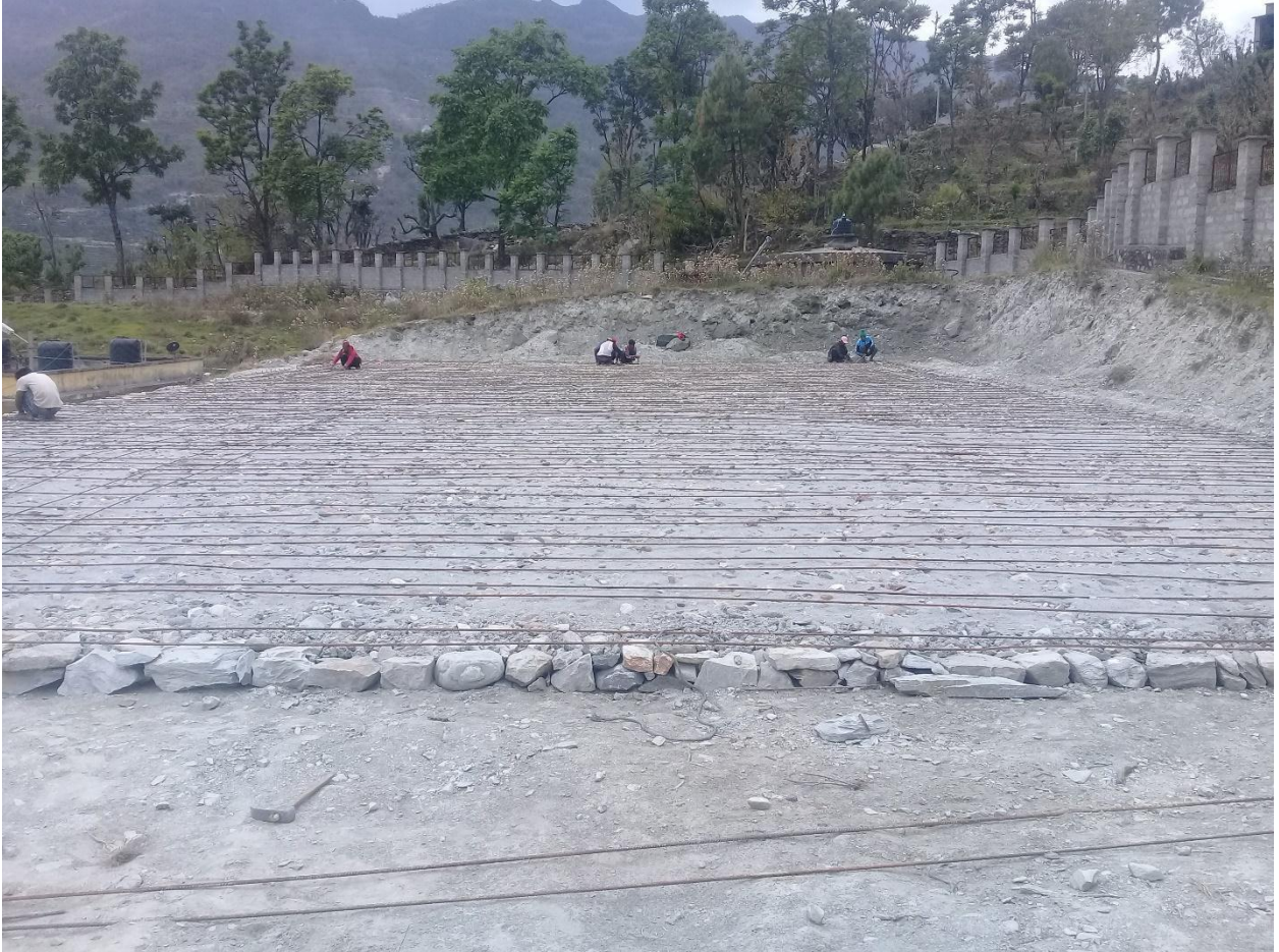
Fig:- Basketball court foundation work being carried out inside camp area
