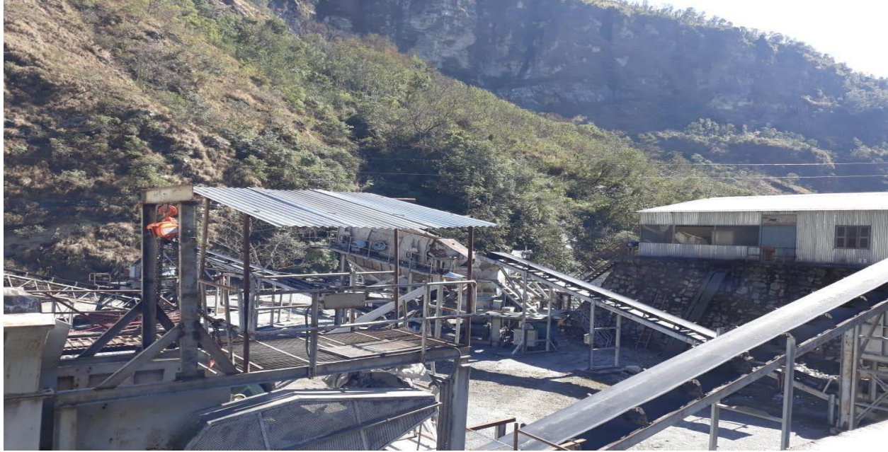
Fig:-Crusher plant installed at Chamare
