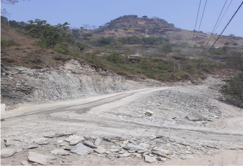
Fig:- Access Road leading to Power house
