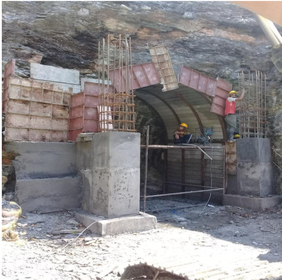
Fig:- In-site work progress at Adit-2 portal face.
