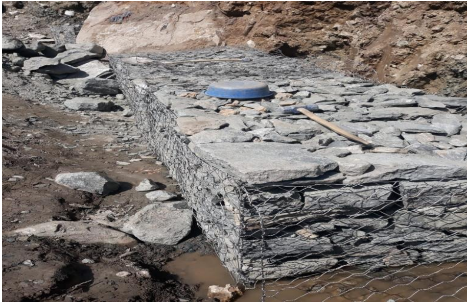
Fig:- Gabion work being done adjacent to project access road.
