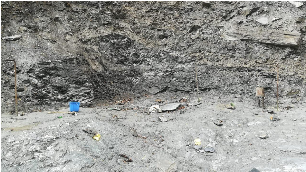
Fig:-Installation of rock anchors at left abutment of Steel through Bridge
