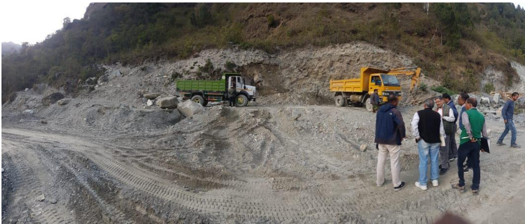
Fig:-Site clearance at Powerhouse
